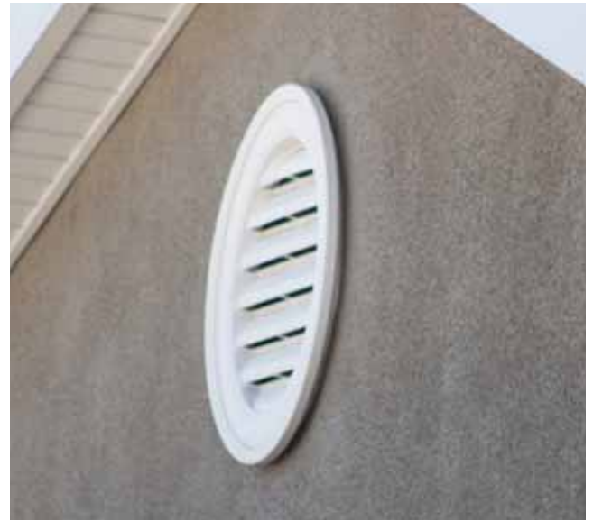
Round Gable Vent on stucco surface
